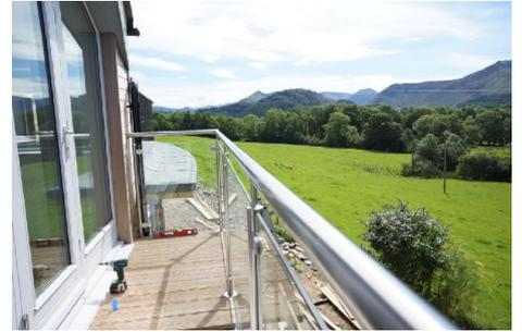
facing away from the road, horizontal timber cladding was applied. This gives the property a sleek modern finish, especially when coupled with the stainless steel and glass balcony. The large 3.6m tall windows, which were installed prior to delivery, capture light and let it flood into the main living space.
